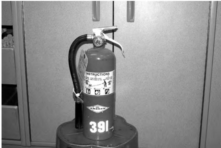
Figure 5-10 Portable extinguishers are marked to indicate what type of fire they should be used on.
